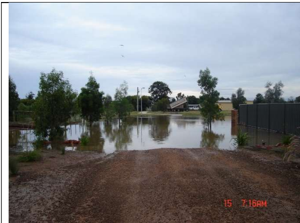
Photograph 1 – view east across the north end of the Black Street retarding basin
