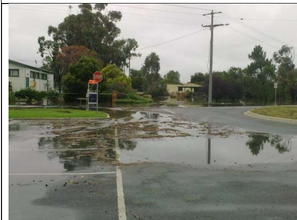
Photograph 5 - Entry road into General Store carpark from Hickey Road
